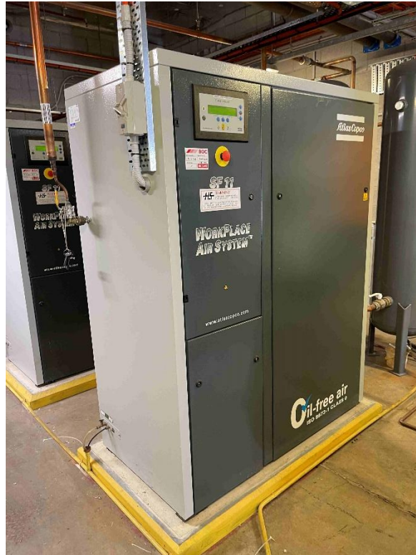
Photograph 15 – Medical Air Compressor in Plantroom
