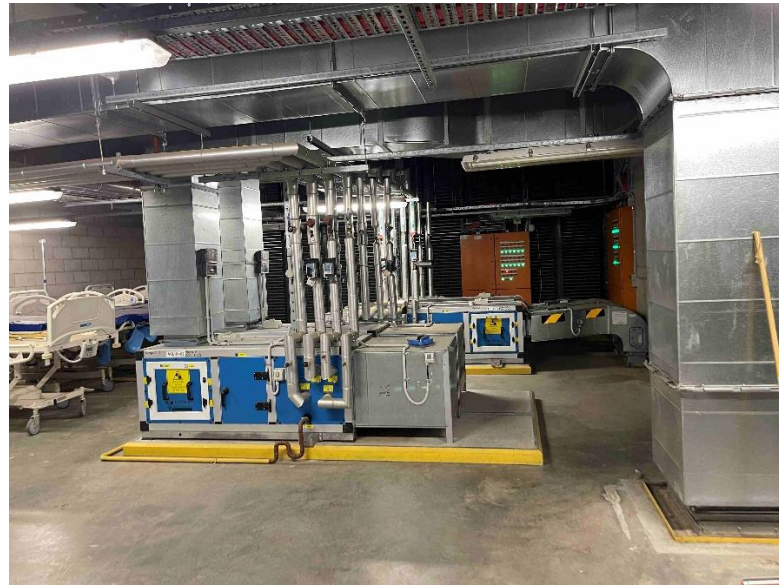
Photograph 11 – Fan Coil Units
