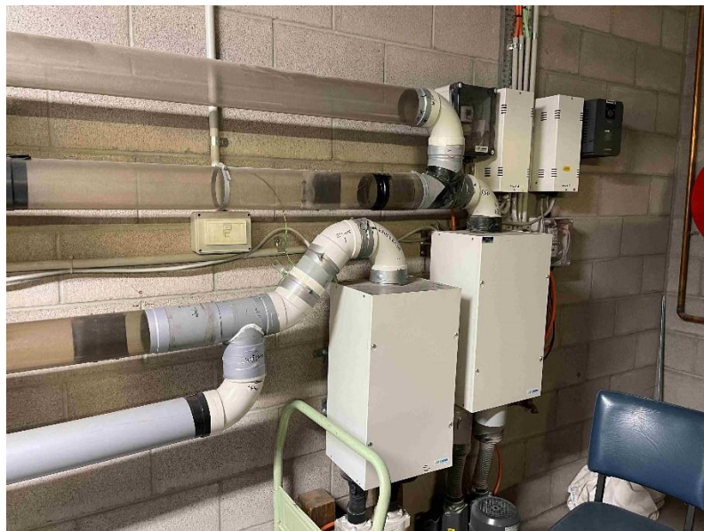
Photograph 12 – Pneumatic Tube Distribution System
