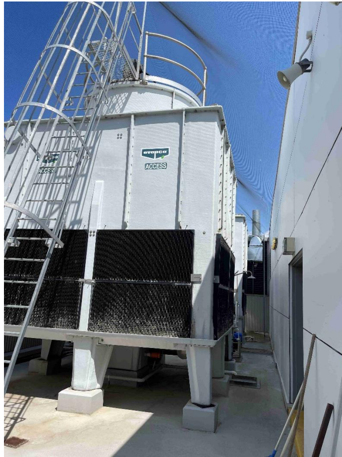
Photograph 7 – Cooling Towers
