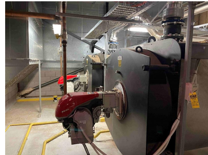
Photograph 9 – Gas-fired heating hot water generators
