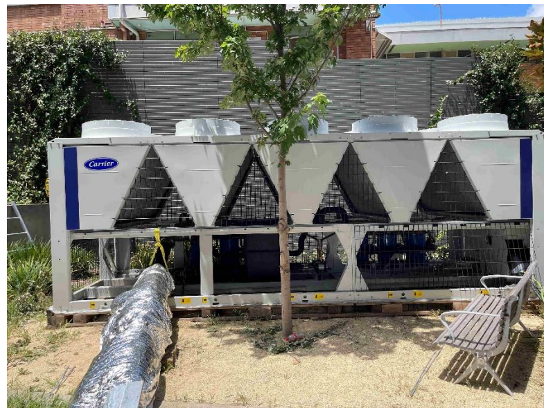
Photograph 8 – Temporary Air-cooled Chiller
