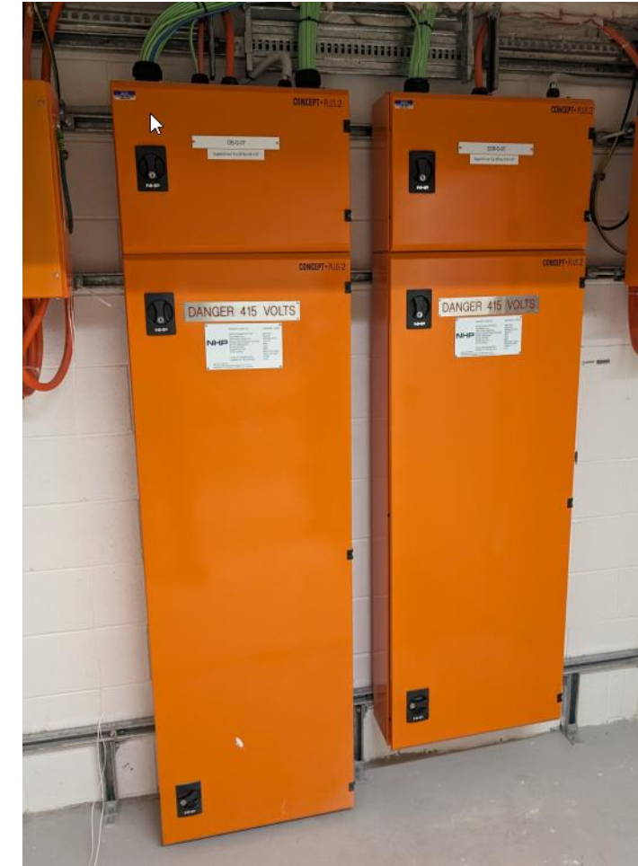
Photograph 16 – Existing Distribution Switchboards DB-G-07 & EDB-G-07
